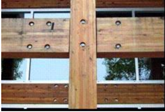
Fig. 1: Example of a bolted beam-column connection with slotted-in steel plate
