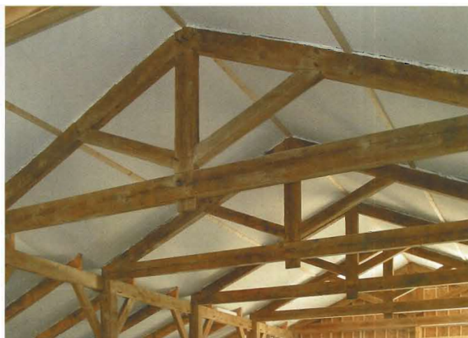
Fig. 17. Typical modern kingpost truss with diagonal web members to support rafters. White oak 6x12 rafters and tie beams span 30 ft.
